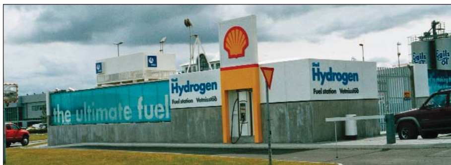
Fill 'er up. Reykjavik's lone hydrogen station, which manufactures the fuel on site by splitting water molecules, can fill a bus with pressurized gas in 6 minutes.
